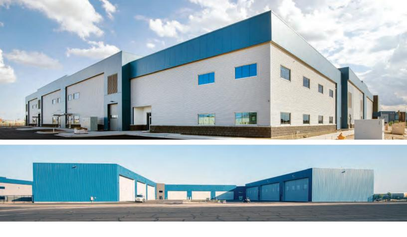
Success of early teamwork was clear with step one of designing a hangar — the door. "The door drives the structure," said St. Clair. "We were involved with the door selection, considering implications that each door can have to the structure, all equating to dollars and time. Nucor and district sales manager Joe Mellody were very integral in helping provide the architect and owner direction — a big part of the money savings early on."
