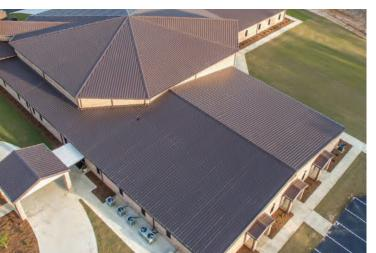
Nucor Building Systems' Loc Seam-90 and Loc Seam-360 Roof Systems are structural standing seam vertical rib roof panels that are perfect for architectural requirements in today's marketplace.
