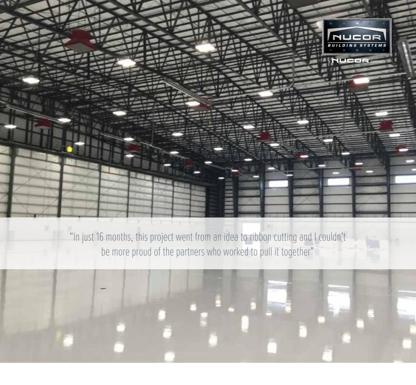
Production began in July of 2014 at Nucor Building Systems' Utah division. The hangar boasts a clear span width of 362' 4'' – the largest span in the Pacific Northwest region in a pre-engineered metal building – and is 365' in depth.
