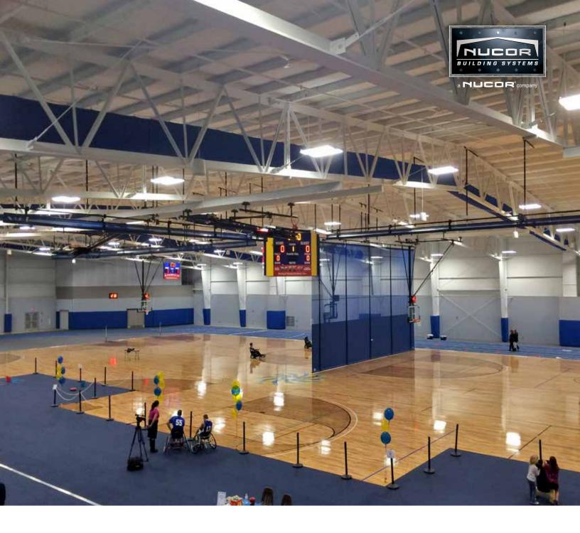
The main structure is a 75,600 sf gable symmetrical clear span at 200' wide with 83" deep TrussFrames. It contains a new field house, which includes a partial mezzanine utilized as a 230 meter track along with four regulation wheelchair basketball courts with digital scoreboards, and two massive divider curtains. A roof beam support holds basketball hoops in place to allow for minimal floor space obstruction.
