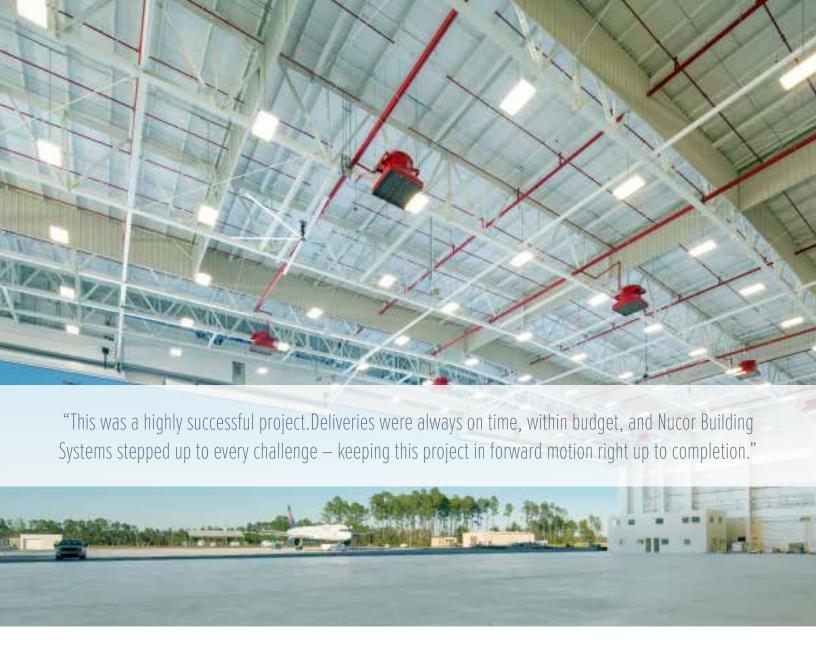
by the open fascia system that is nearly 15'0" in height. It also features Nucor Wall Lites which allow for natural lighting to be dispersed throughout the building's interior as well as energy conservation. Several draft curtains were installed to aid as smoke barriers along both sidewalls and front endwall.
