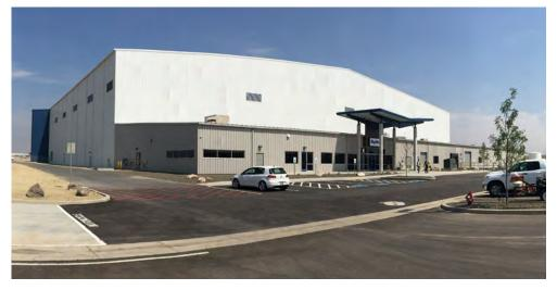
overhead clearance of 62'. The solid web columns supporting the TrussFrame rafter system are an imposing 10' in depth. Nucor Building Systems worked with hangar door manufacturer, Norco, to integrate their product seamlessly with the Nucor building, and meet the needs of the customer. The building's exterior is finished with Nucor's CFR<sup>™</sup> standing seam roof system, and Nucor Reverse Classic<sup>™</sup> wall panels.
