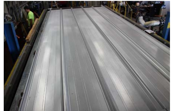
Installed Panel (Fig.6)
