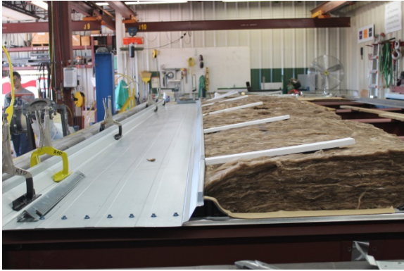
Installation with Clamp (Fig.1)
