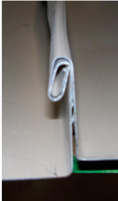
Finished "Vise Lock 360" Seam
