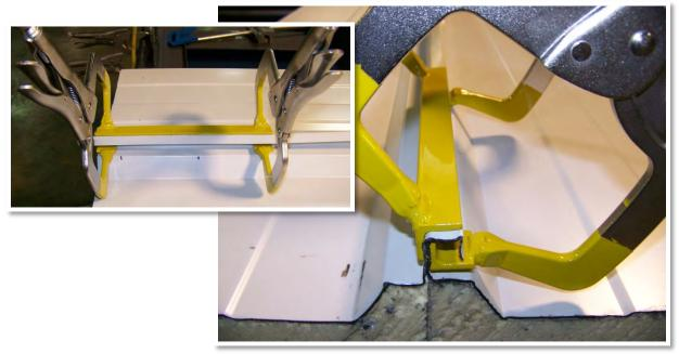
**STEP 3:** Place the provided hand crimper on top of the clamp <u>and</u> panel, between the two handles. Move the hand crimper's action handle its full range of motion to complete the crimp. This crimp will secure the two panels together.
