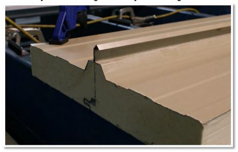
**STEP 2:** Place the Seam Clamp on the seam, flush against the end of the panel. This will force the top sheet down and nest the two panels together tightly.
