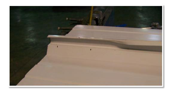
**STEP 6:** Apply the Roof Seamer over the hand crimped portion as shown, giving special attention to the direction the machine will travel after power is supplied. This will be indicated on the top or sides of the power unit. **The Roof Seamer is designed to run from the Ridge to the Low Eave.**
