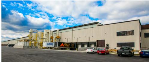
The exterior of the building is finished with Nucor Classic Wall™ Panel and uses a Nucor CFR™ Standing Seam Roof System.
