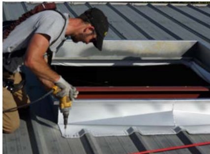
3. Install roof curb.
