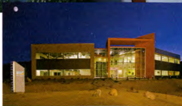
The 95,000-square-foot Schluter Systems Distribution Center and Training Facility in Reno, Nev., consists of a 75,000-square-foot warehouse constructed with pre-engineered steel and a 20,000-square-foot office constructed with structural steel. Among the many energy-efficient elements incorporated in the project include ceiling skylights installed throughout the warehouse, offices and atrium providing extensive natural daylight resulting in 75 percent of the employees working under natural light. Miles Construction, Carson City, Nev., was the builder.
