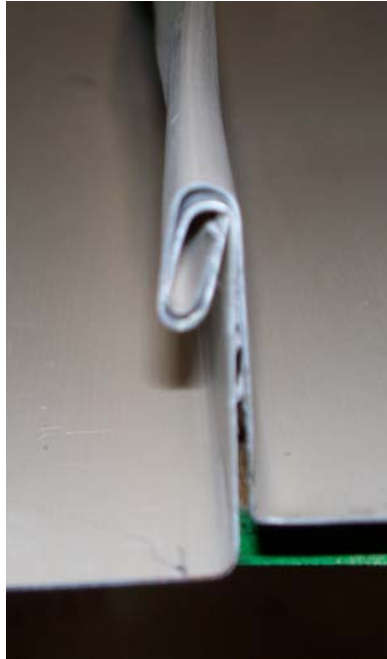
Finished "Vise Lock 360" Seam
